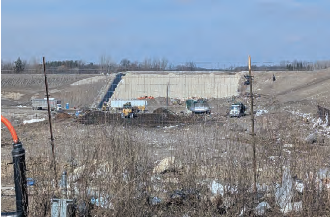
View North across Phase 4
