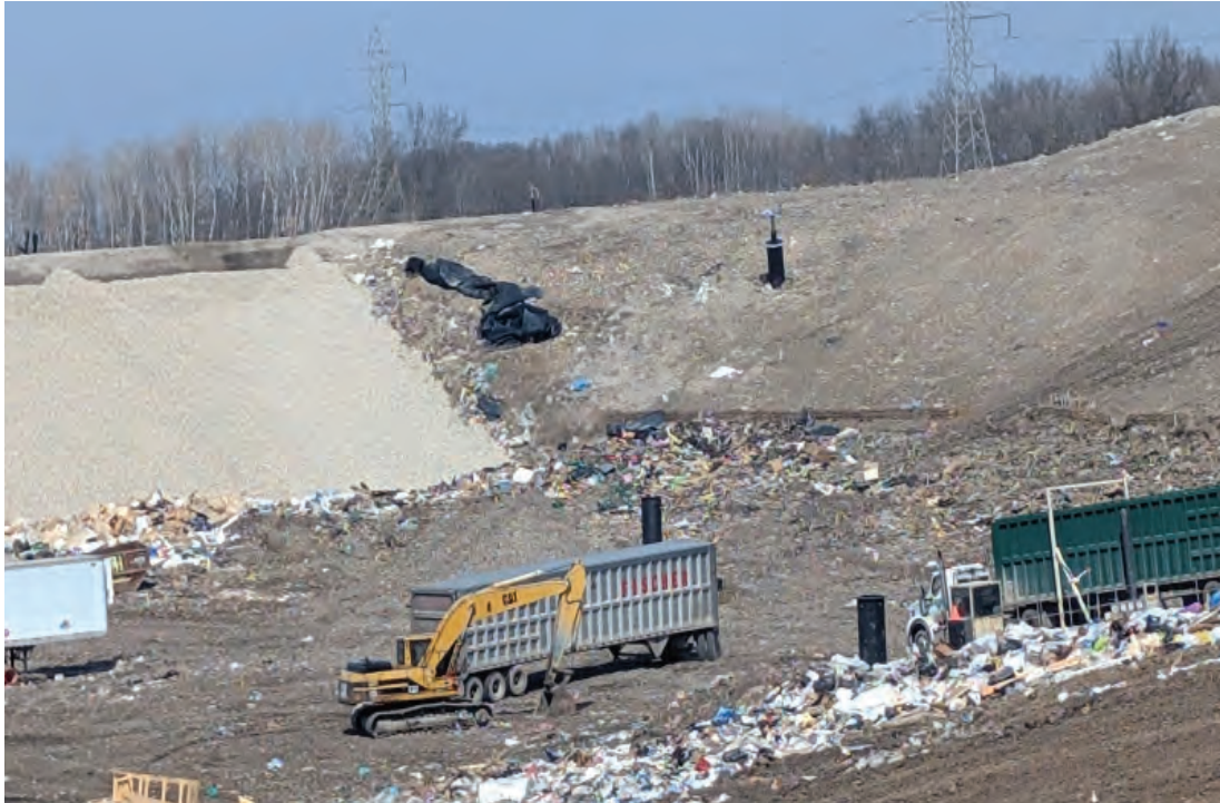
North end of Phase 4, note two wells installed
