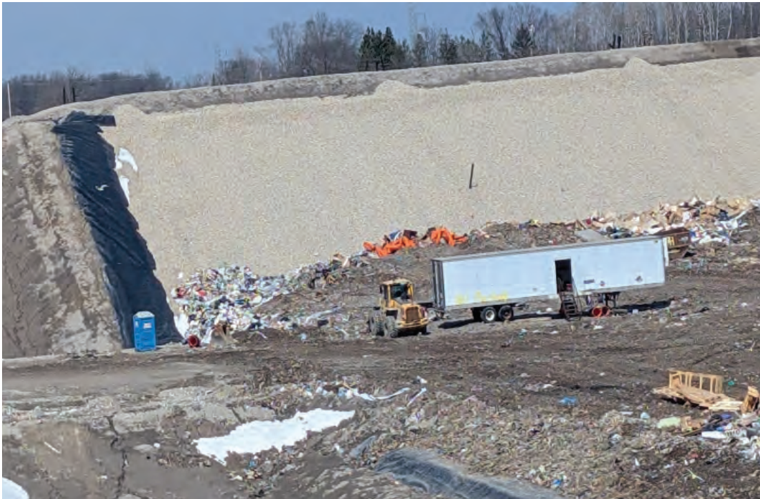
Access to Phase 4 across rain flap
