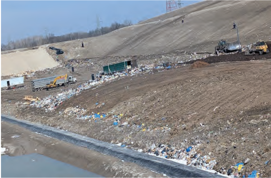
Rain flap on West edge of Phase 4, note water elevation in temp sed pond
